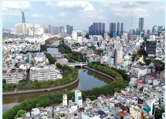
Urban infrastructure along both banks of the Nhieu Loc-Thi Nghe canal in Ho Chi Minh City__Photo: Thanh Vu/VNA
